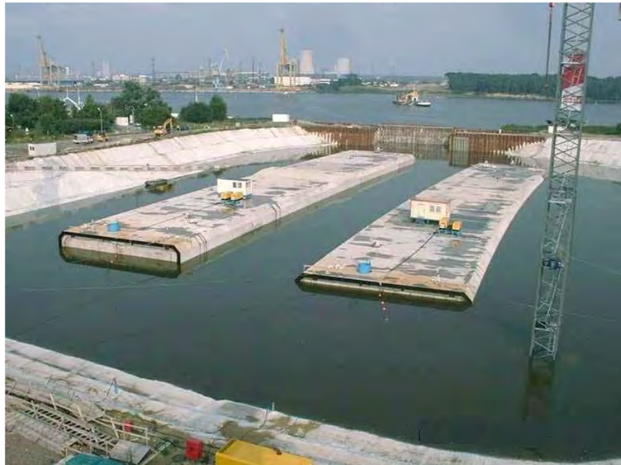
Figure: Tunnel elements floating in construction dock
