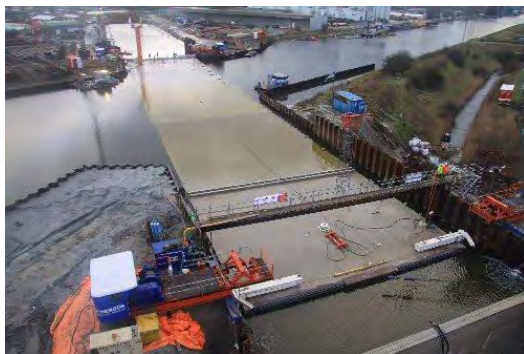
Figure: The immersion process in progress
