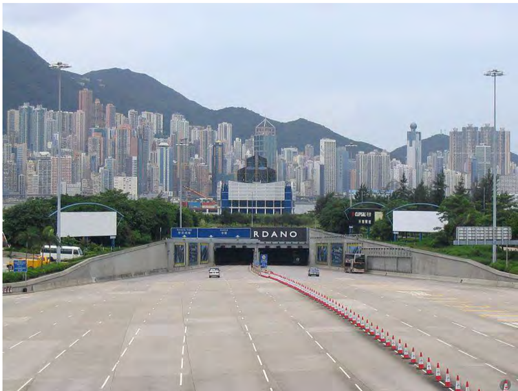
Figure: tunnel in operation (source: internet)
