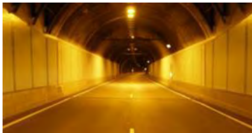
Figure view of western tube of the Westerschelde tunnel.
