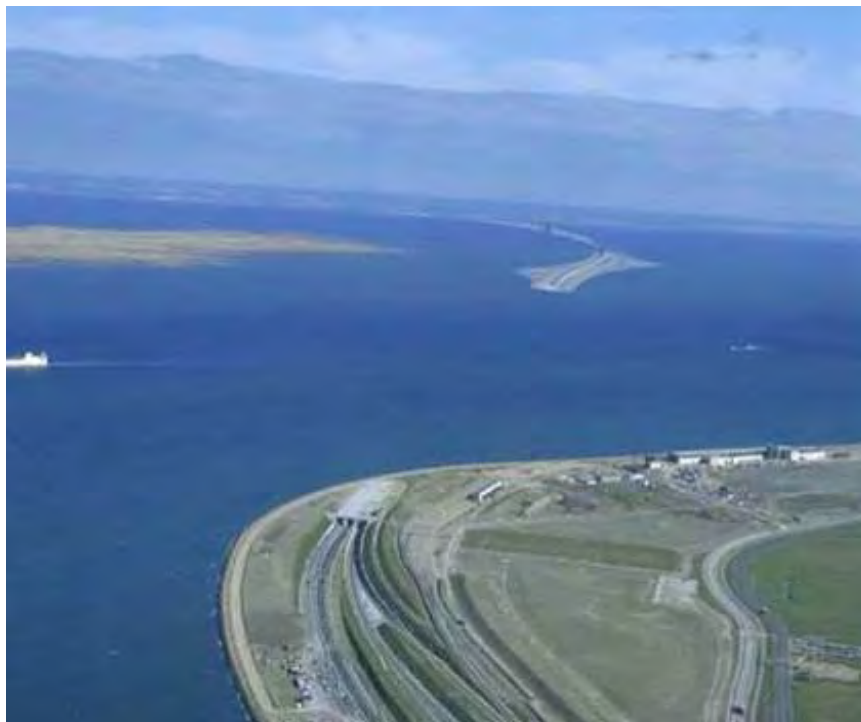
Figure: tunnel entrance & artificial island
