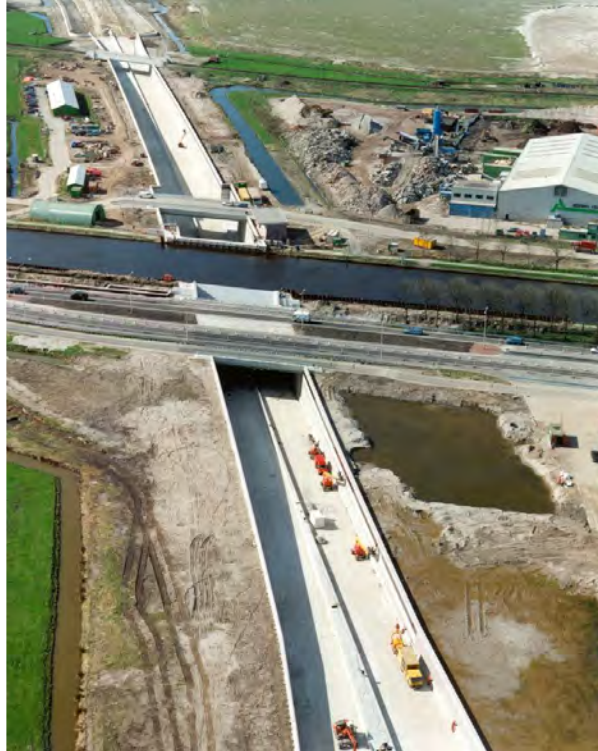
Figure: Aquaduct under construction
