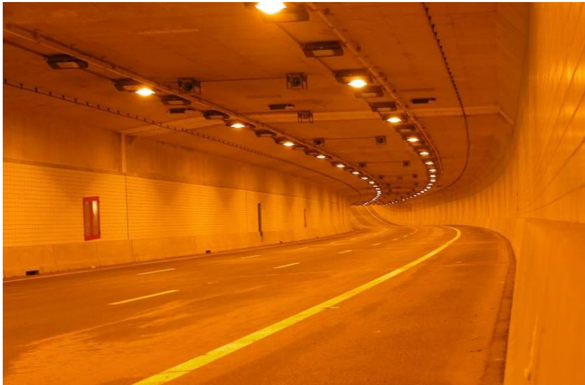
Figure view of tunnel tube with 3 lanes of the Thomassen tunnel.
