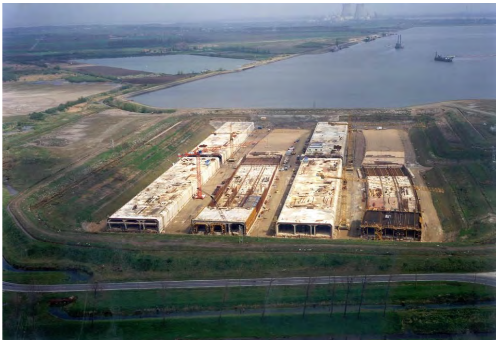
Figure: Tunnel elements in construction dock (Verrebroek dock Antwerp)
