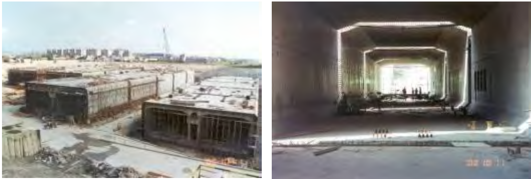
Figure: Tunnel elements under construction
