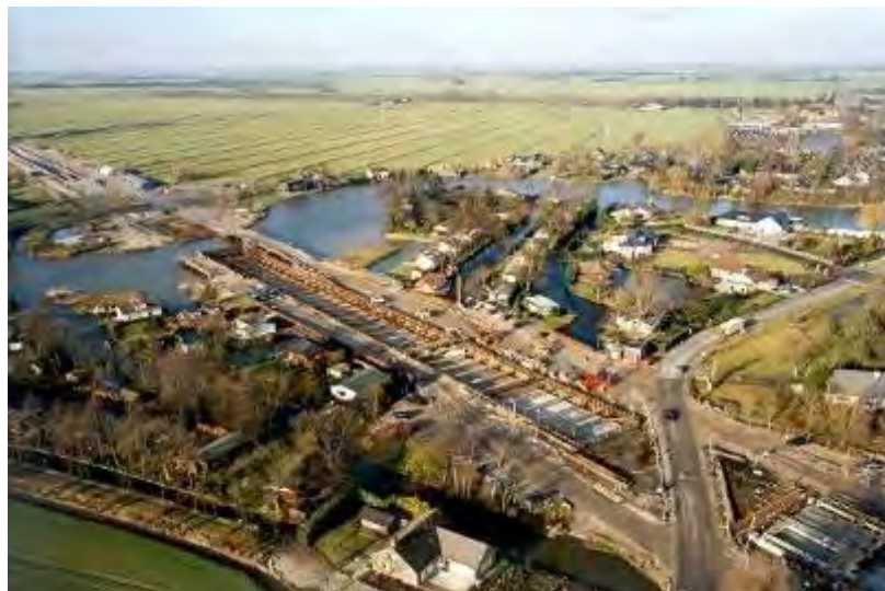
Figure: Tunnel under the Giessen under construction
