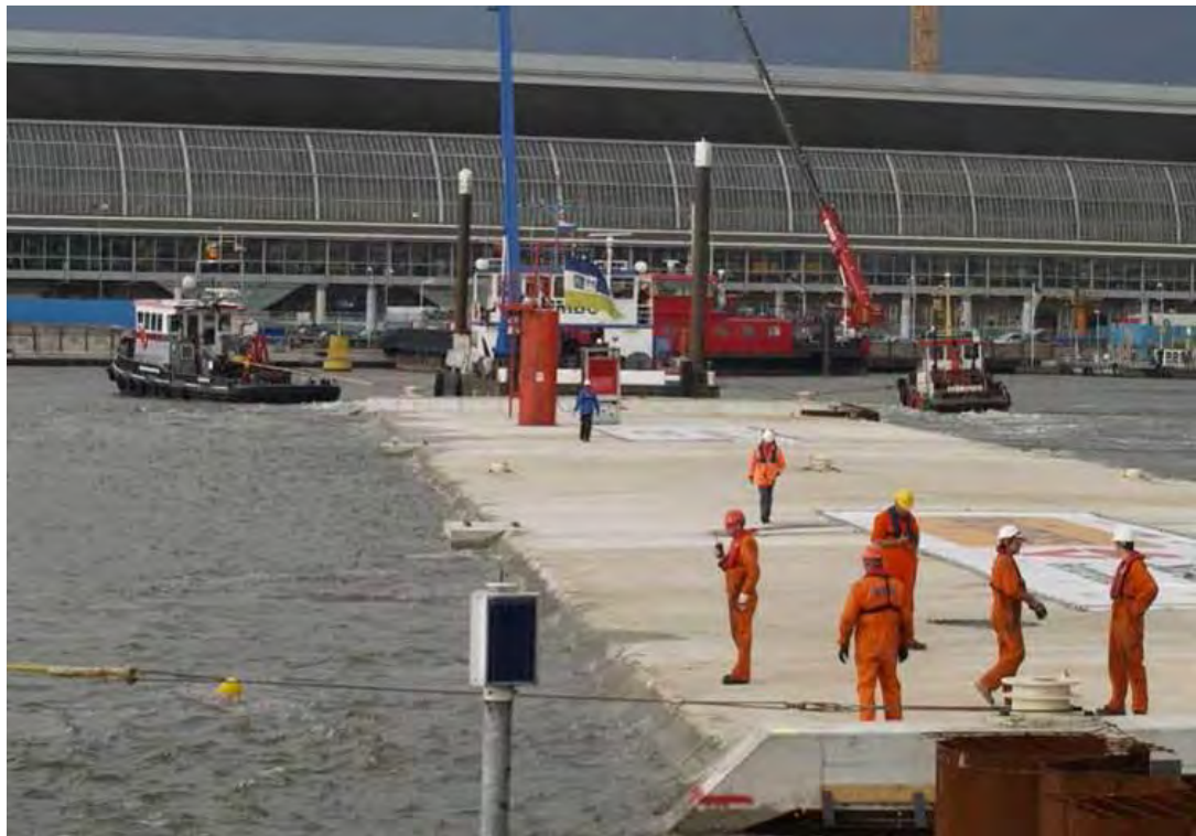
Figure transportation and immersion of tunnelement.
