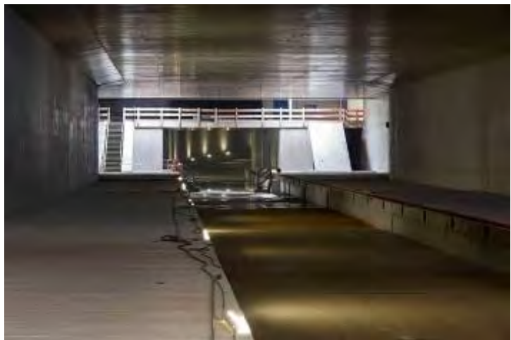
Figure: Main civil works for Station completed
