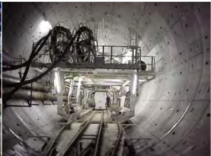
Figure: tunnel lining
