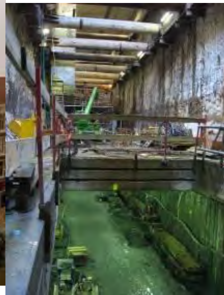
Figure: Station under construction
