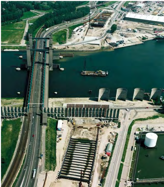
Figure: Tunnel under construction
