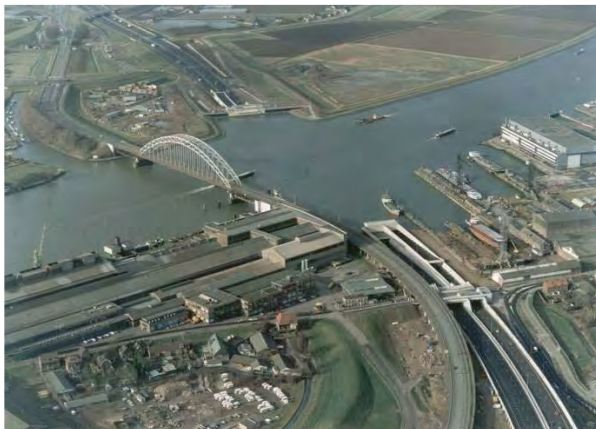
Figure: Tunnel under the river Noord
