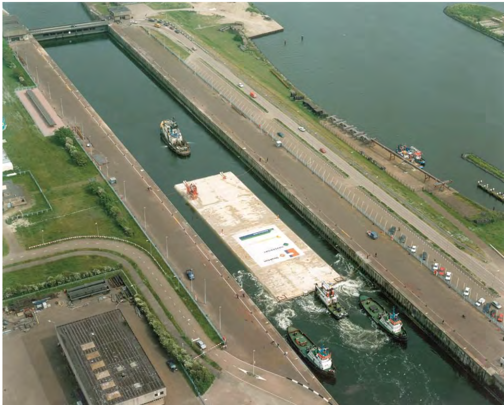
Figure: transport tunnel elements
