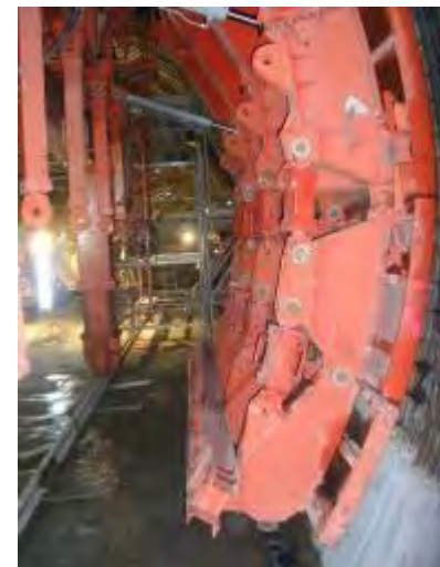
Figure: inner lining formwork
