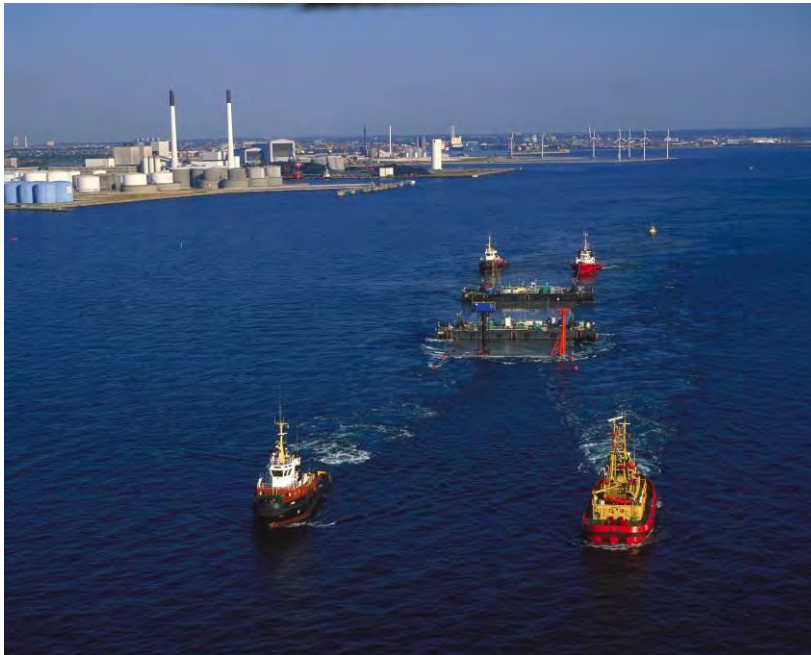
Figure: Transport of tunnel element
