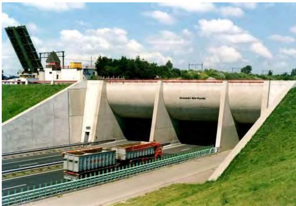
Figure: The Aqueduct in operation
