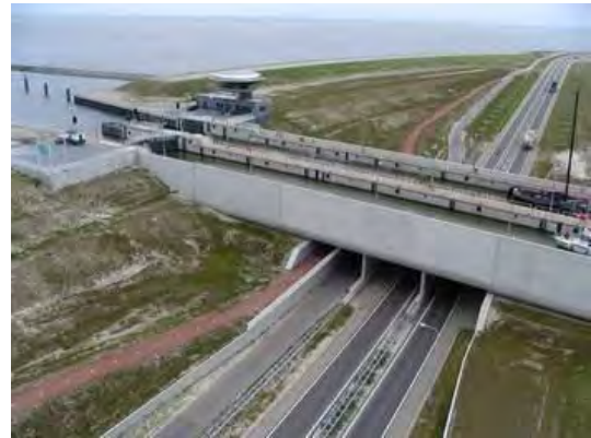
Figure: Naviduct completed (source VBK Groep)
