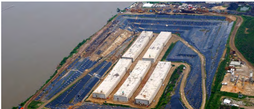
Figure: Tunnel elements under construction
