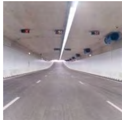
Figure: Tunnel interior
