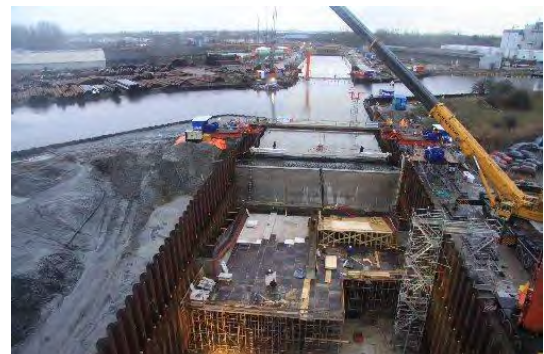
Figure: The element in place
