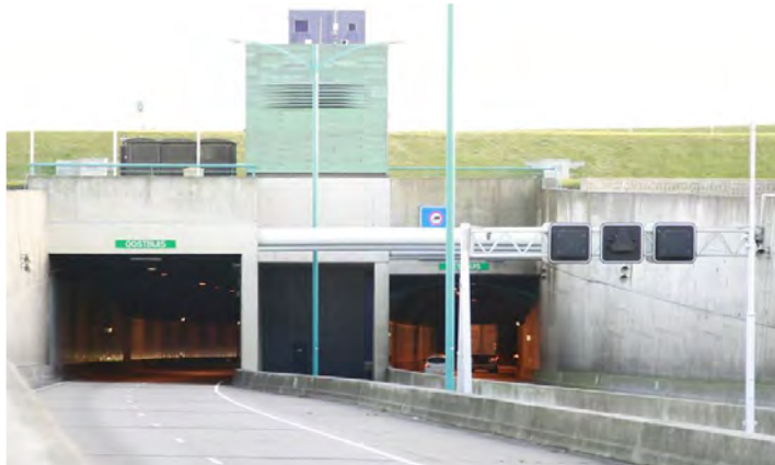
Figure southern entrance of the Westerschelde tunnel.
