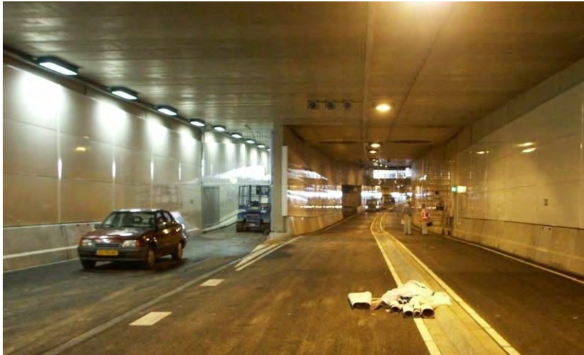
Figure: Junction on the Southern side inside the tunnel tube.
