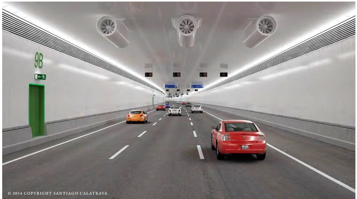
Figure : Interior of the tunnel
